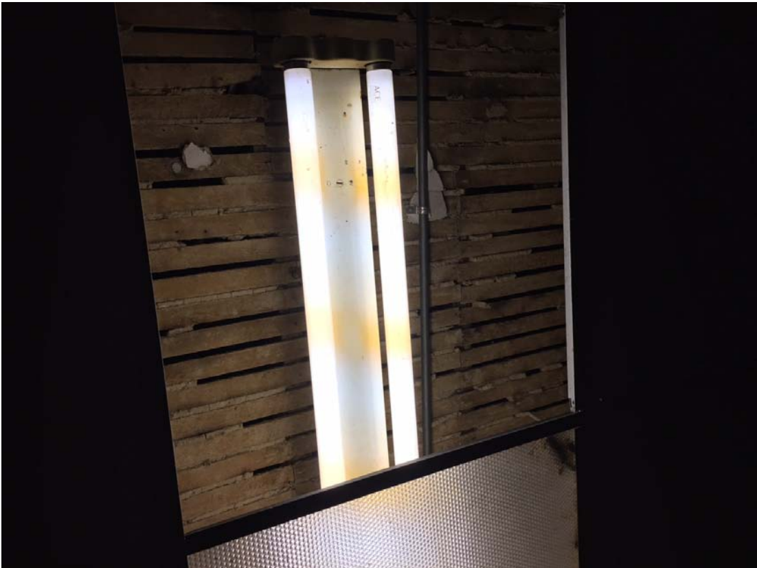
View of ceiling, second floor.
