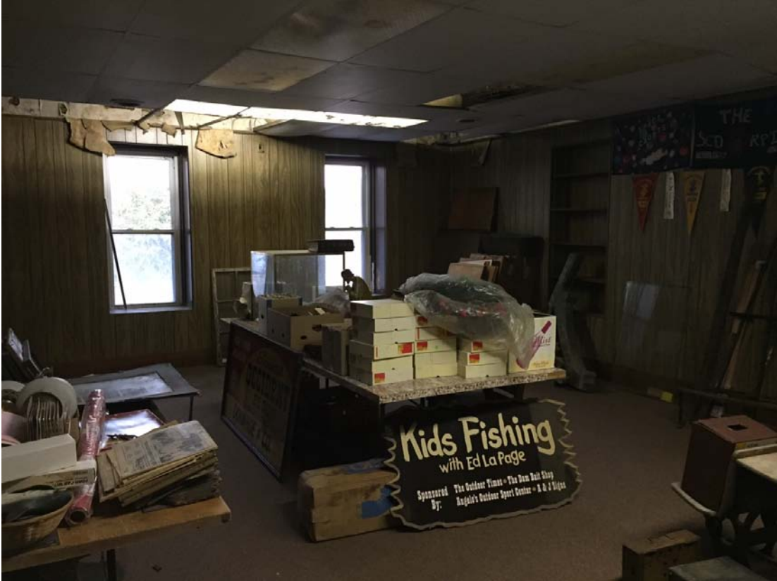
View of second floor interior.
